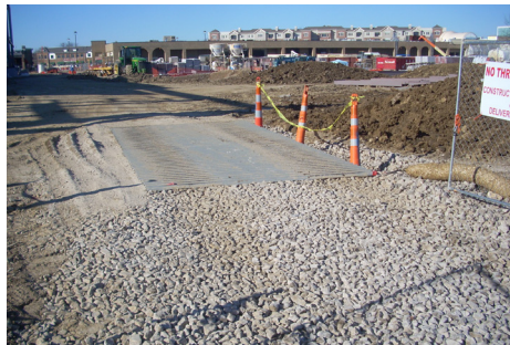
This construction entrance has added a rumble strip for additional debris collection.
