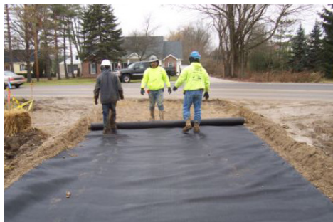
Geotextile helps prevent the stone layer from sinking into the ground.
