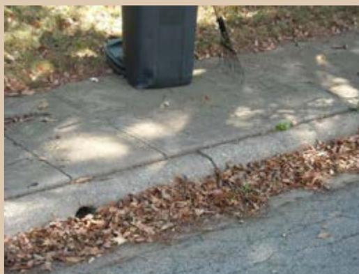
The leaves that have accumulated along this curb can impact water quality if flushed to a nearby stream or pond and should be removed. The small circular opening in the curb is where roof gutters and basement sump pumps discharge, and if clogged can lead to property damage via gutter blockages, basement flooding, and ice dams
