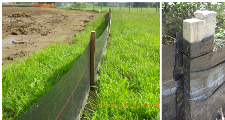
Above are two GREAT examples; proper silt fence installation along the contours WITH a vegetative buffer strip, and the proper way to join two sections.
