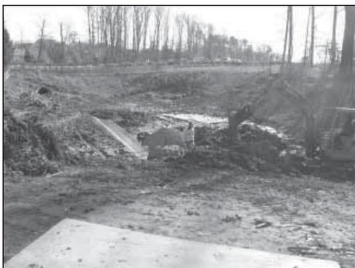
*Removing sediment from stormwater facilities can be a considerable expense. Look for opportunities to reduce the amount of sediment entering the pond from the surrounding drainage area.*
