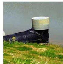
*Riser - forces the water level to rise above outlet before water leaves the pond*
